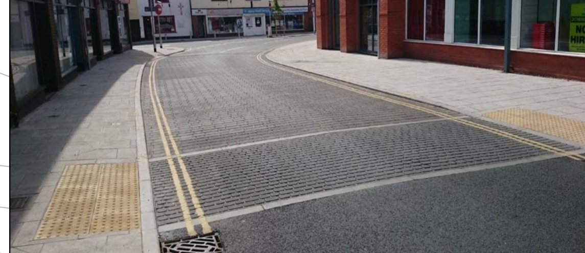
IMAGE 2: IMPRINT SURFACING USED TO REDUCE VEHICLE SPEEDS BY VIBRATION AND CREATE A CONTRASTING SURFACE TO VISUALLY IDENTIFY AN AREA WITH HIGHER PEDESTRIAN TRAFFIC, TIVERTON HIGH STREET
